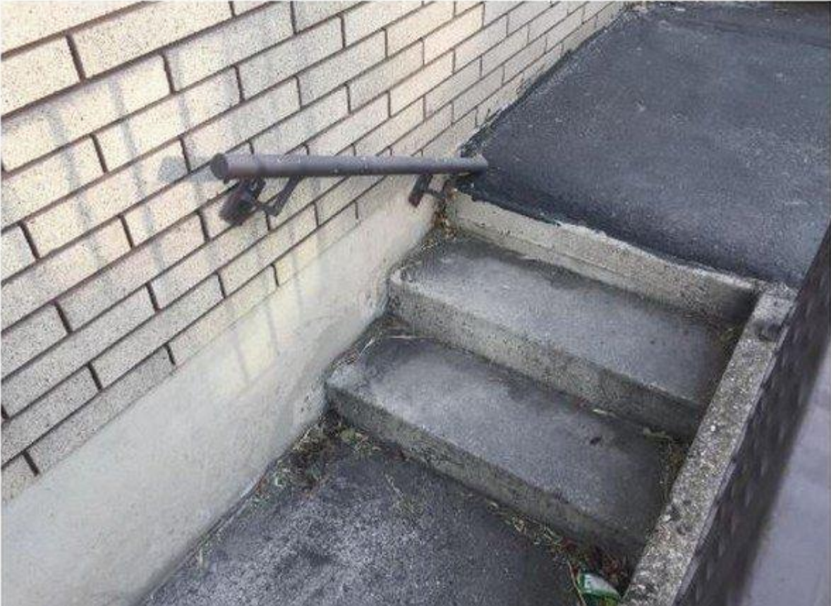
Installed the new handrail, Boss.
